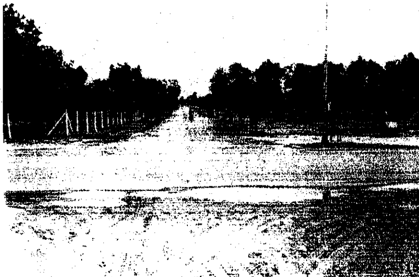
Fig. 13-15 Photographs of Prahlad Nagar area showing the new roads under construction
